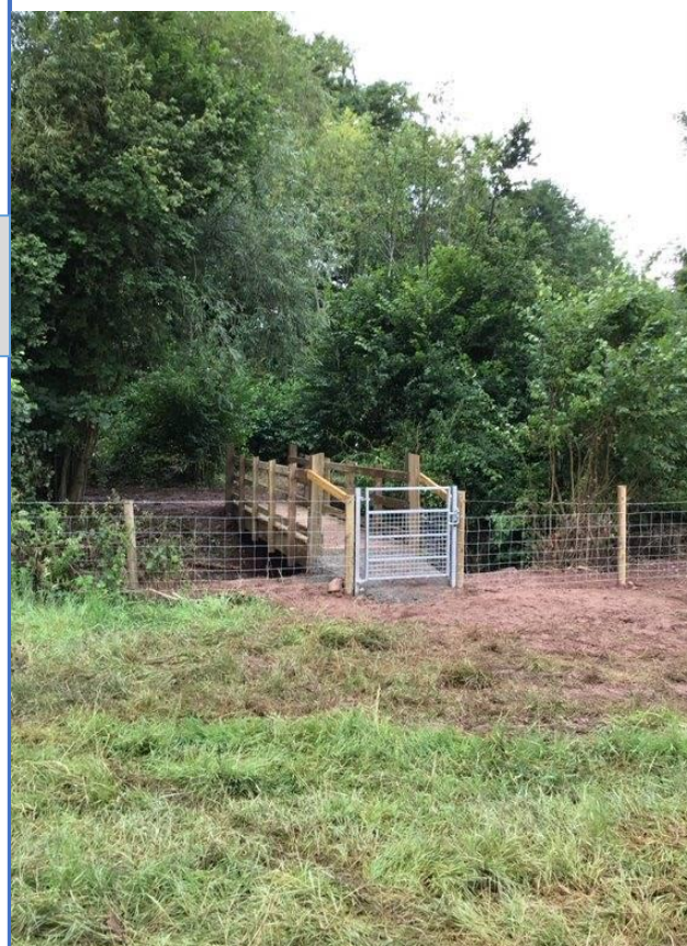
Kingstone Footpath Bridge
