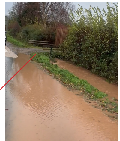
Culvert across ditch blocking flow
