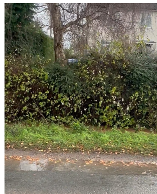
Ditch after culvert empty
